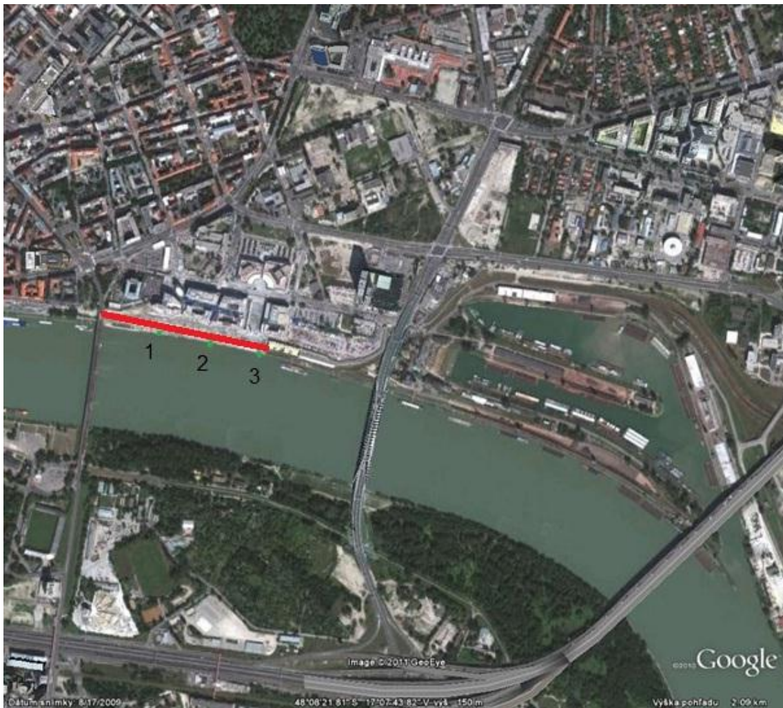
Fig.1: Top view of three bridges in Bratislava.
