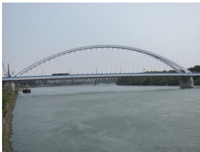
Fig. 4 View point C
